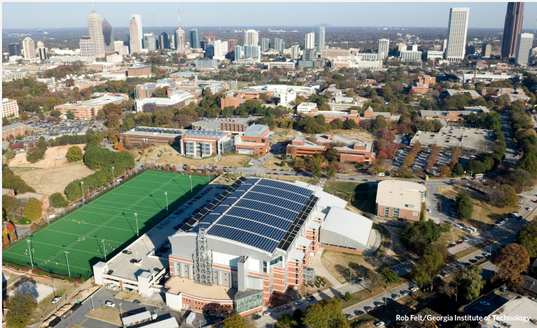
Rooftop Solar Array at Georgia Tech's Campus Recreation Center.
