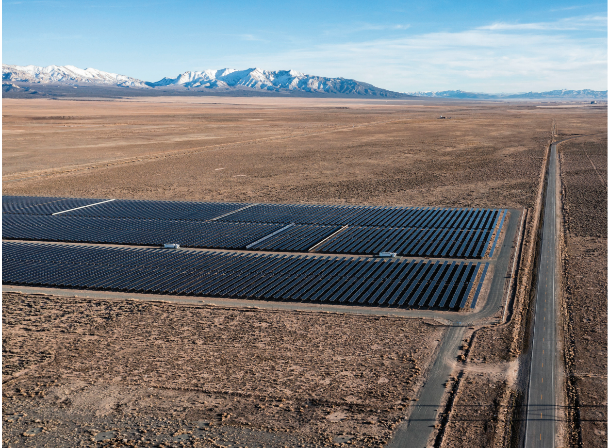
Solar power, collected with photovoltaic arrays like this one in the Utah desert, makes up more than 68% of the state's renewable energy mix. Jon G. Fuller/VW Pics/Universal Images Group via Getty Images
