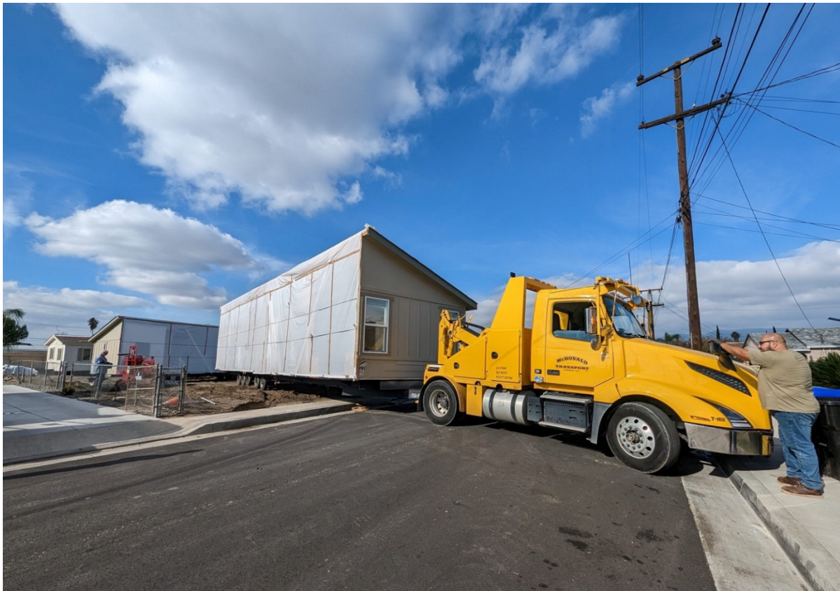
The second half of a NPHS-developed factory-built home being sited on a lot in San Bernardino. The NPHS team noted that for infill development, narrow streets and small lots can present a challenge for the efficient siting of homes. Where space is especially limited, a crane may be required to maneuver the home into place, adding significant expense to the project cost.
