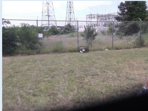
Weymouth 1 – Fore River Energy Center
